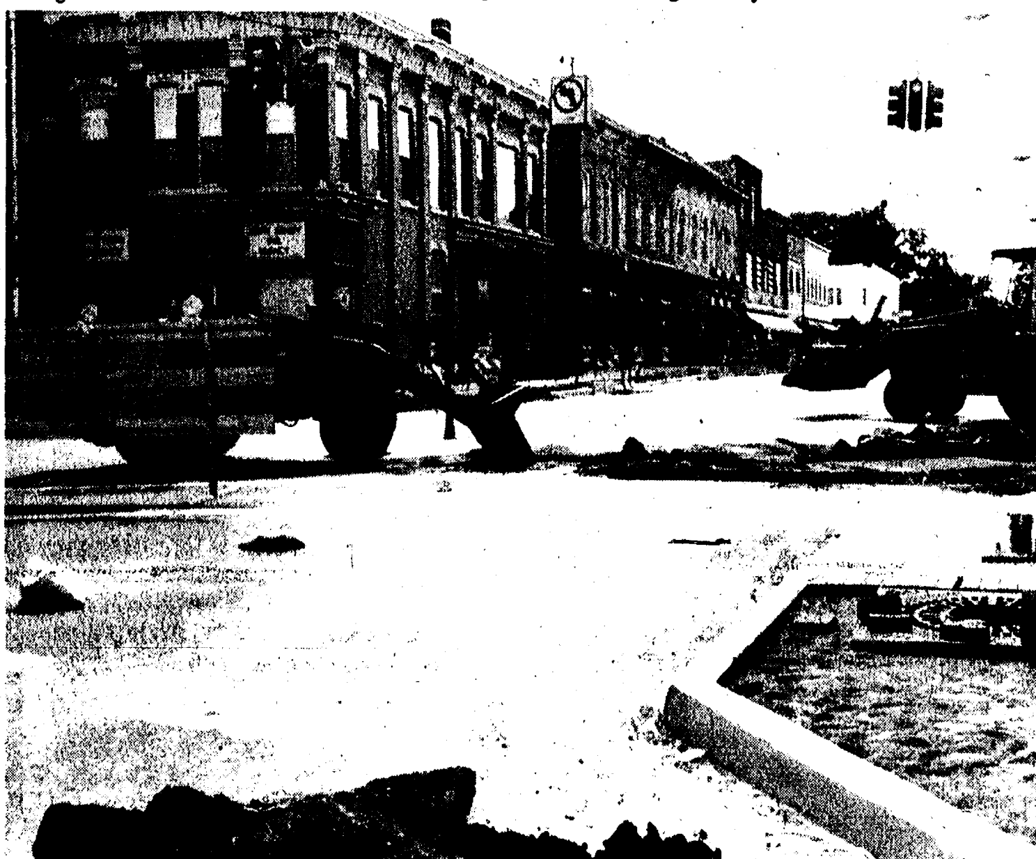
ELECTRICAL CABLES will be buried under Main St. as part of the Downtown Development Authority project. However, as workers cut across the road on the north side of W. Middle St. they found a washed out area under the road, caused by a cracked stormwater pipe. There was plenty of cause for concern because the affected area of road has no support. The sewer will have to be repaired and the village plans to install a manhole there.
